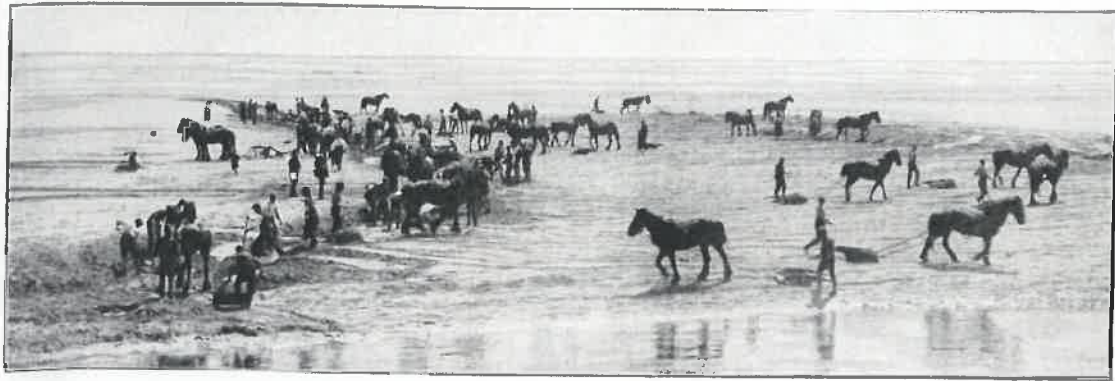
AS ALLIANCE UPON MANY DOZENS MEN, WITH 10 HORSES VOLUNTARILY ENGAGED AT KARAMEA SELSON, IN THE CUTTING OF A CHANNEL TO STRAIGHTEN AND DEEPEN THE RIVER AND IMPROVE THE HARBOUR. J. M. Hawes, Photo
